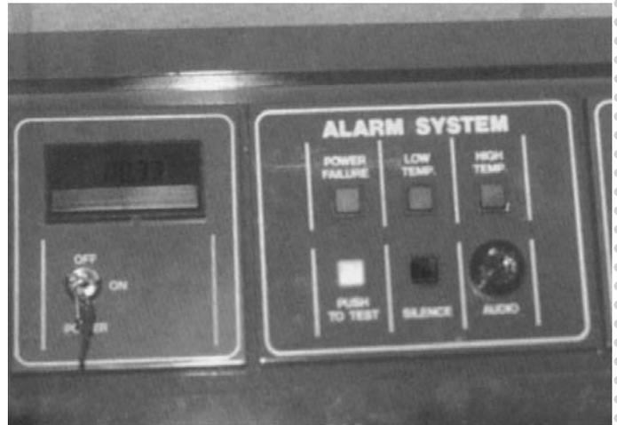
**Figure 2** An alarm system that calls you or a guard if there is a temperature malfunction.
